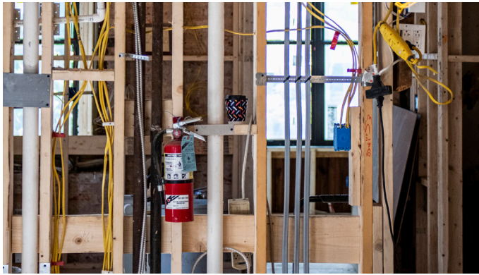
Repairs and upgrades continue inside. All photos by Eric Bond/FCNL.
